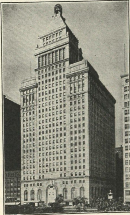
STRAUS BUILDING • Chicago Graham, Anderson, Probst & White Architects
