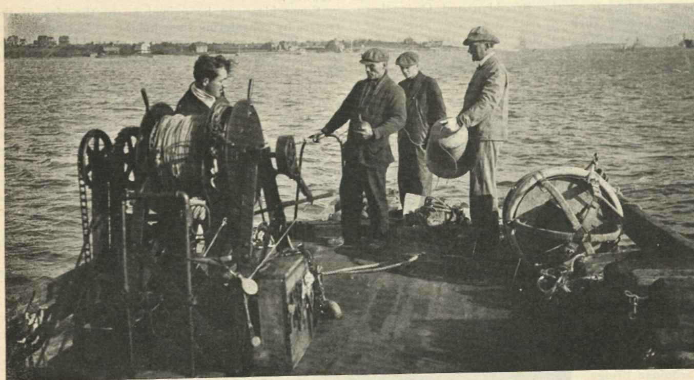
Preparing the Wire Drag.
