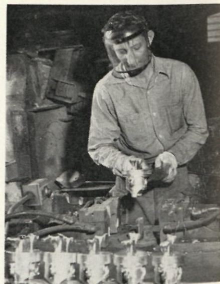
REMOVING PISTON FROM MOLD IN THE FOUNDRY. NOTE HAND LADLE BEHIND WORKER.
