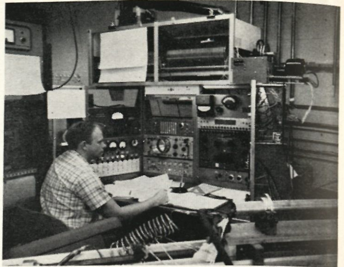
JOHN KEITH, GRADUATE STUDENT IN PHYSICS, TAKING DATA FROM THE CONSOLE OF THE BETA-RAY SPECTROMETER.
