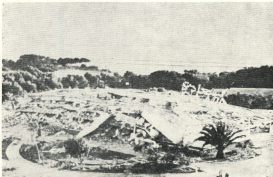
Figure 1b: Saada Hotel After Earthquake. (1,40)
