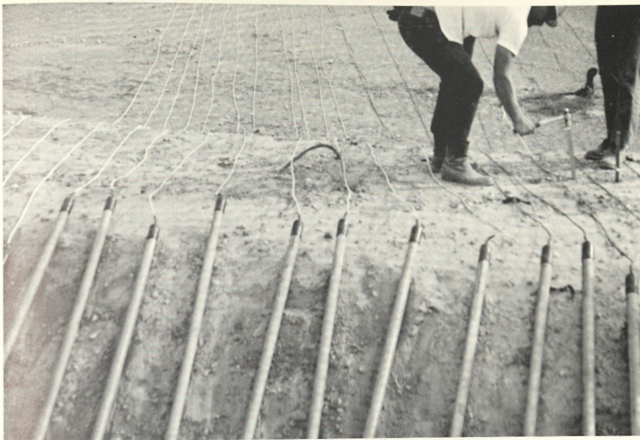
Figure 11. (above) These are iron anodes being layed out for easy access just before lowering into the deep-well ground bed.
