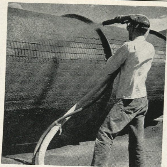
To Harness a River ----- pipe protected with CLINTON WELDED WIRE FABRIC
