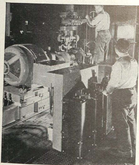
Graduate students conduct performance tests of centrifugal pump units.
