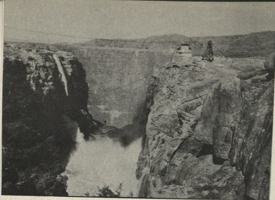
PATHFINDER DAM. Located on the North Platte river, this masonry arch-gravity type dam stands 214 feet high.
