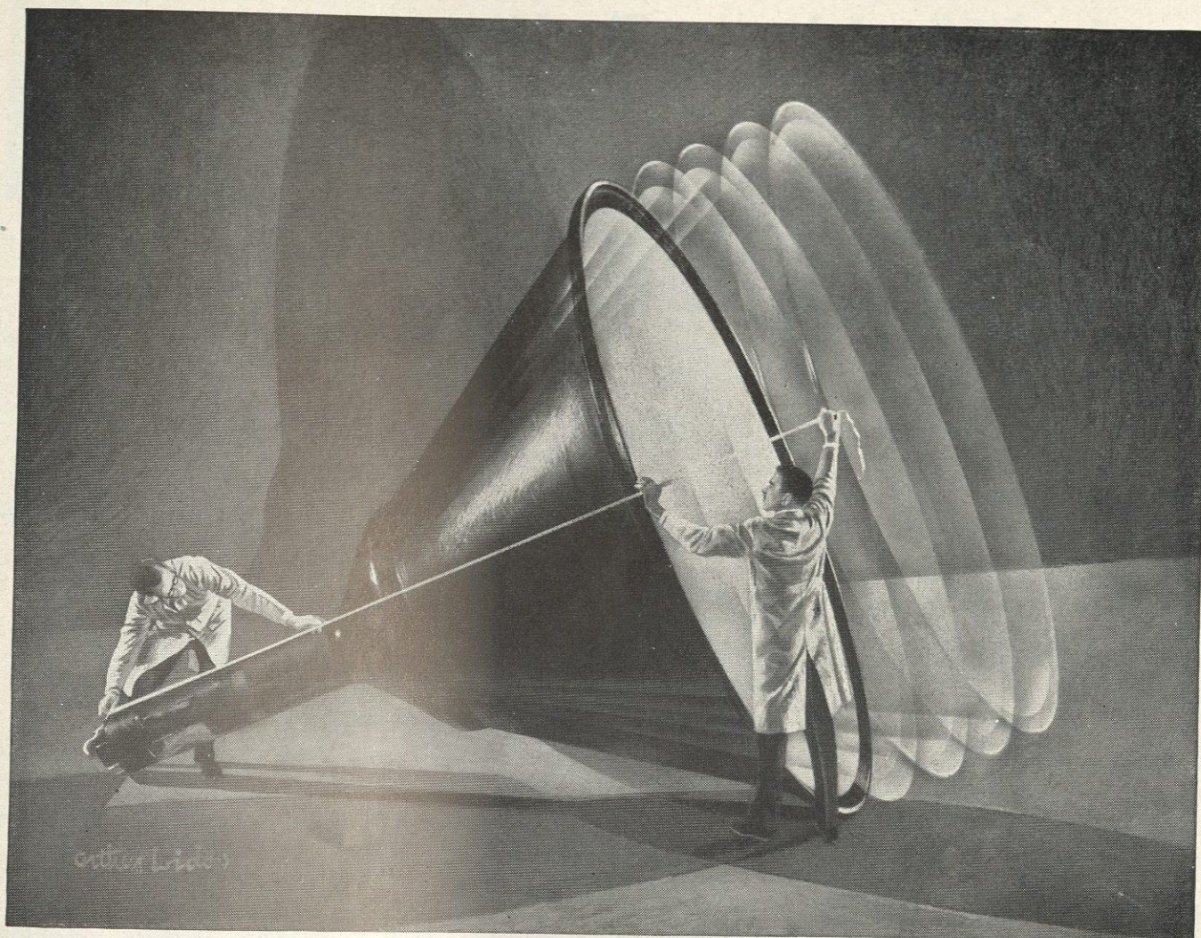
New and shorter big screen 16-inch kinescope developed by RCA scientists.
