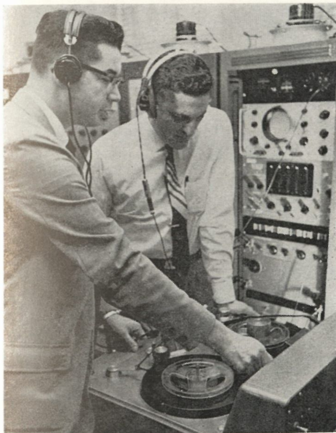
Dr. Louis J. Gerstman (left) and Dr. J. L. Kelly, Jr., of Bell Telephone Laboratories, listen to a tape recording of synthesized speech which was produced by an electronic digital computer. The computer is fed, on punched cards, the names of speech sounds which make up an English sentence. It processes this information and produces synthesized speech in digital form on a magnetic tape. This tape is converted—on the machine behind Kelly and Gerstman—into a \frac{1}{4} -inch magnetic tape suitable for playing on an ordinary tape recorder.
