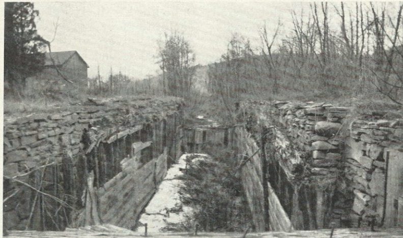
This view of a lock section of the Delaware and Hudson Canal gives a good impression of the stone work which has endured for over 100 years as silent testimony of the skill of the builders.
