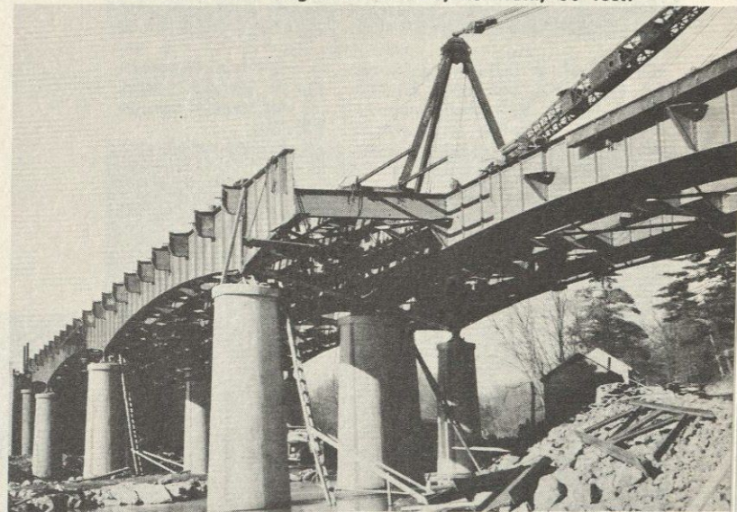
—Courtesy American Inst. of Steel Construction Placing a deck girder span on permanent abutments performed by a traveling derrick near Cincinnati Union Terminal.
