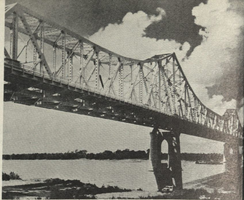
—Courtesy American Inst. of Steel Const. The O. K. Allen Bridge, Louisiana. An example of the through cantilever type structure.
