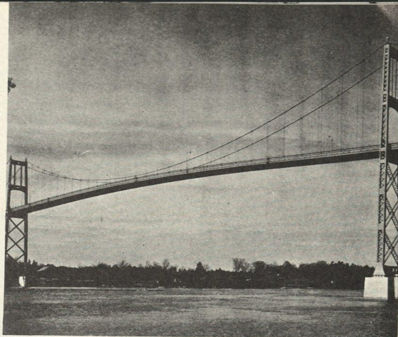
—Courtesy D. B. Steinman Connecting the U. S. Mainland to Wells Island, Canada, is this spectacular suspension bridge with a main span of 800 feet.
