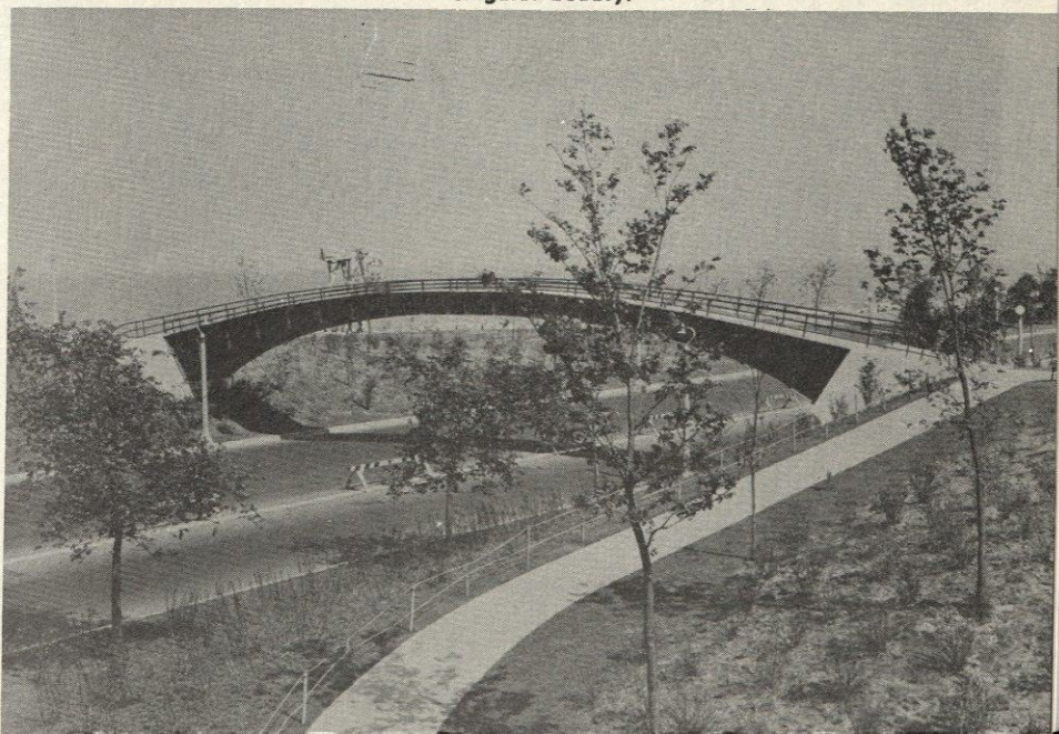
—Courtesy American Inst. of Steel Const. This pedestrian bridge, Burnham Park, Chicago, Ill., is an arched girder bridge of singular beauty.
