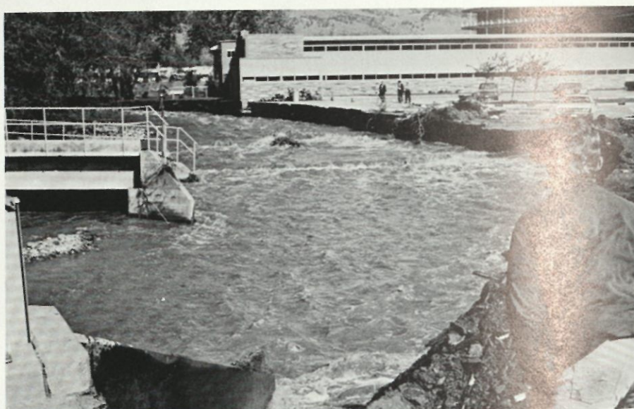
Photograph looking west from 28th St. bridge in Boulder Colo. shows the extensive damage to a nearby bridge. The bridge was removed a few weeks later. Note that the corner of the building in the background was undercut by flood waters. Photograph was taken a few days after the May 1969 Boulder Flood. DAILY CAMERA PHOTO
