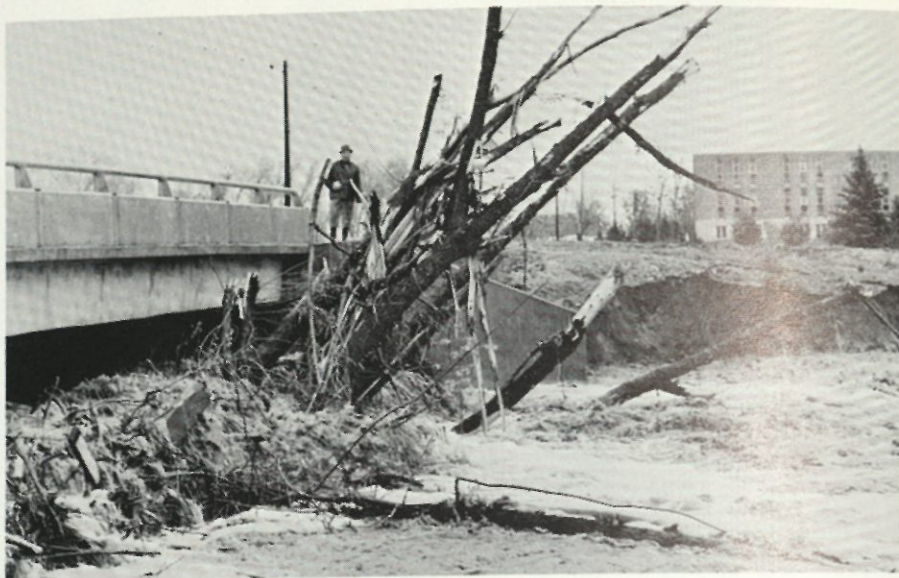
Debris piled under bridges was a major problem during the May 1969 Boulder Flood. Channel improvements required by Boulder's Flood-plain Zoning would help alleviate this type of damage. DAILY CAMERA PHOTO
