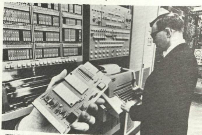
TELEPHONE CENTRAL OFFICE. Invention of the transistor enabled telephone switching systems, which identify, switch and route calls dialed by telephone customers, to be converted from electro-mechanical to fully-electrical switching. The circuit pack (foreground) shows typical packaging of integrated circuits used in electronic switching. This modern switching method is fast, accurate and versatile.
