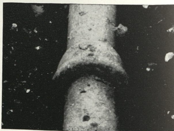
This 123-year-old cast iron water main is still in use in the distribution system of St. Louis, Mo.
