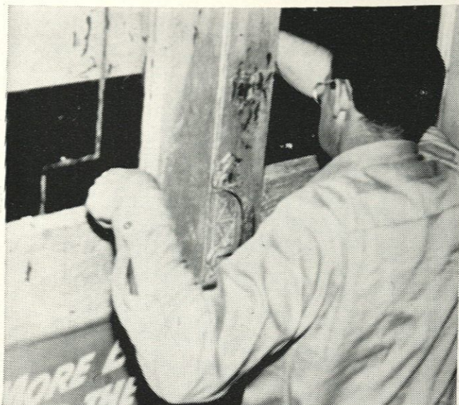
The burglar, after breaking the glass in the door of this grocery store, reaches inside to unlock the door latch. Unknown to him, the building is wired for burglar alarm protection. Tape wiring, as seen above his left hand on the window, was torn and the closed circuit was broken when the window was smashed.
