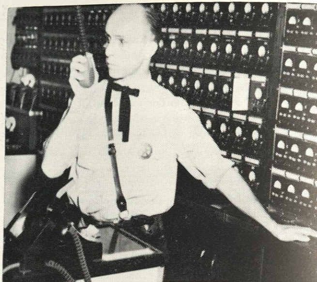
Central station is given a signal that the closed circuit in the building is broken on one of these panel receivers. The dispatcher checks a card and finds that the building was not scheduled to be opened at this time and radios a company patrol truck and the police.
