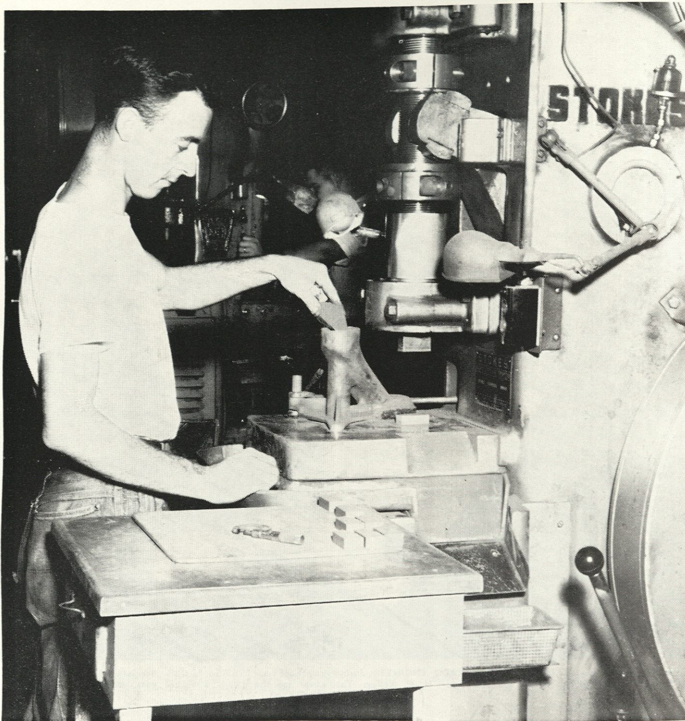
The press operator measures out a quantity of metal powder in preparation for the pressing operation. Note the use of a micrometer, an indication of close tolerances.
