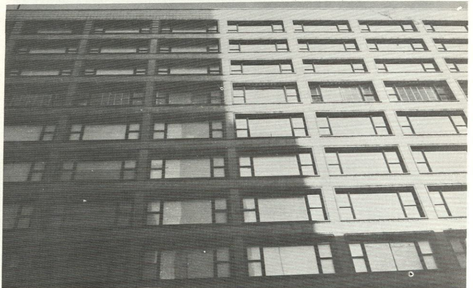
The "Chicago Window" Carson Pirie Scott Building, west face. 1899, 1903–04, 1906. Louis Sullivan.
