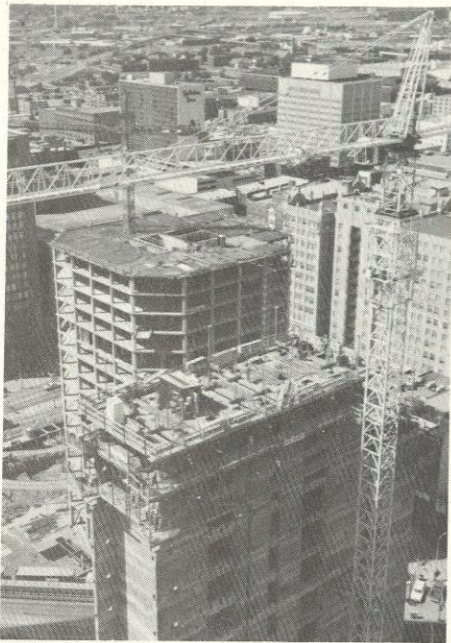
The multiactivity nature of the slipform can be seen in this photo. The fresh concrete is placed in the hoppers atop the platform. The slipform itself is at the second level and the third level is used for welding the structural endpieces to the embedded plates.
