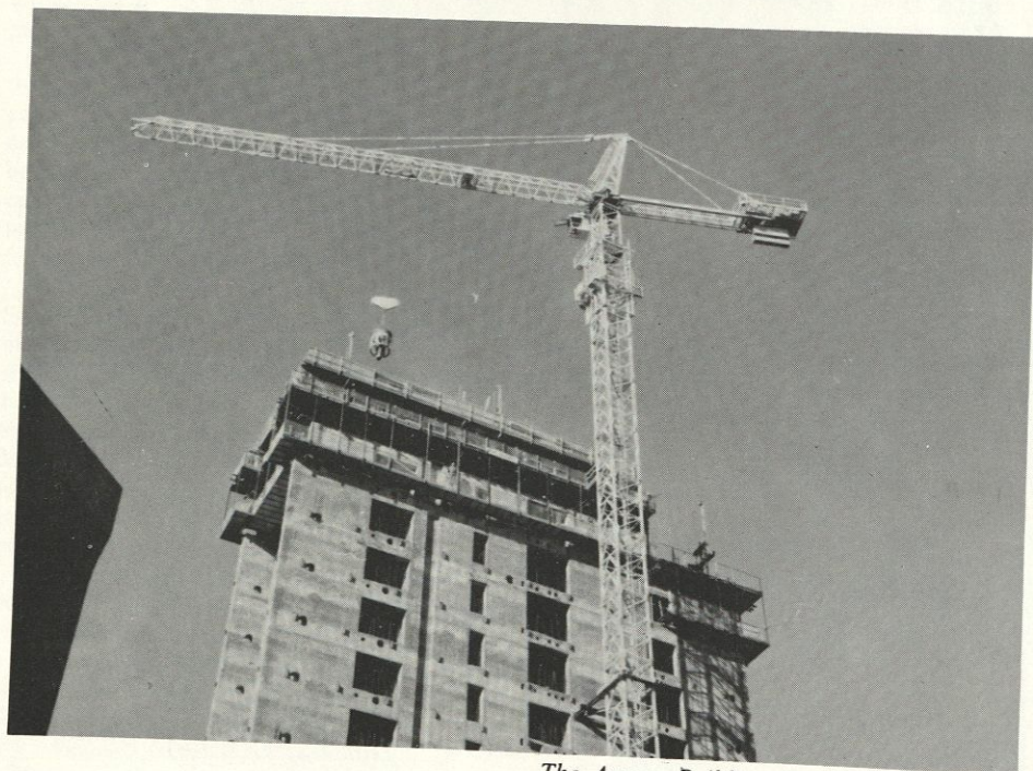
The Amoco Building, currently under construction in downtown Denver, exemplifies the use of concrete slipform techniques.
