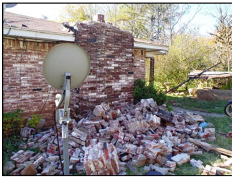
Collapsed chimney from the 2011 Prague, OK M_w 5.7 Earthquake. (Gallucci 2014)
