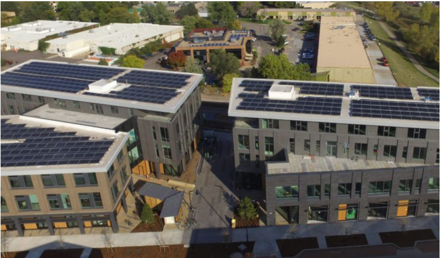
The roof of a commercial complex in Boulder, Colorado, uses an angled mounting design to further optimize the efficiency of photovoltaic cells. ( bouldercommons.com )
