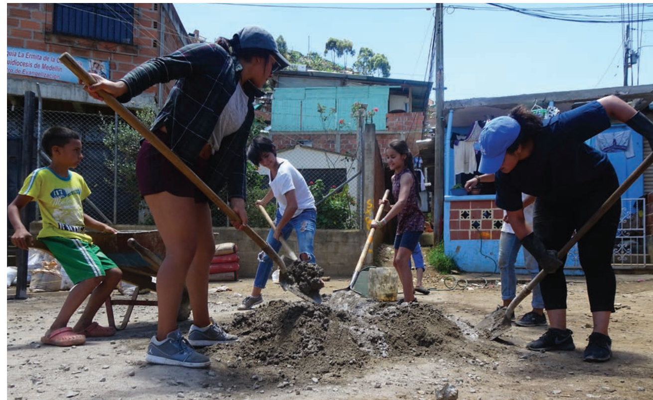
CU Boulder students and community members prepare concrete for a shed foundation in a Colombian settlement. Photo by Jota Samper, CU Boulder
