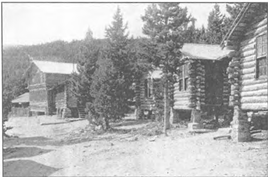
Family cabins (right, Nos. 7 and 9) were built east of the Dining Hall after 1932. (Archives, UCB Libraries)
