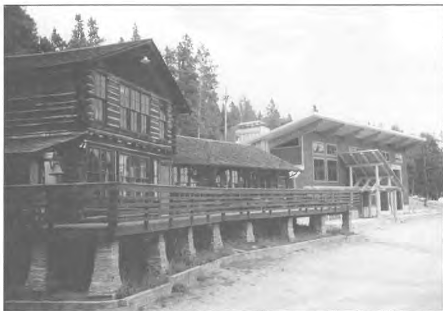
The Dining Hall and new hostel under construction in 1999. (J. Kindig)
