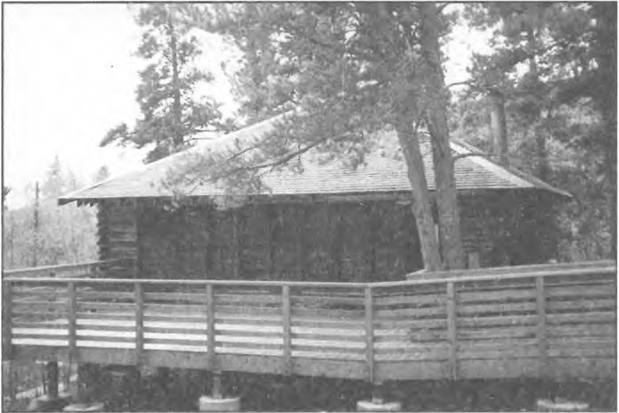
A new ramp and deck have been added to the Megaron. (1999) (J. Kindig)
