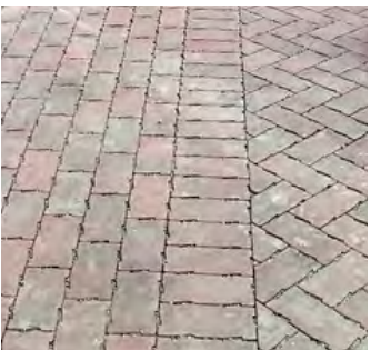
Pervious Pavers at Farrand Field
