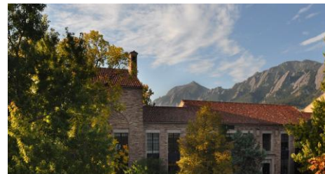
HELLEMS ARTS AND SCIENCES BUILDING
