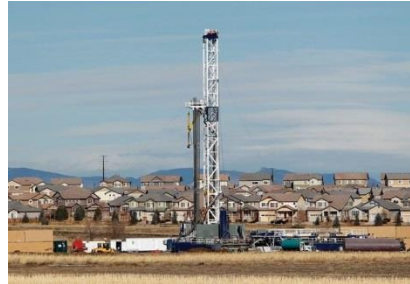
Fig. 4. Drilling rig set up near subdivision in Frederick, CO. 239
