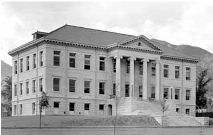
GUGGENHEIM LAW BUILDING , 1909-59.
