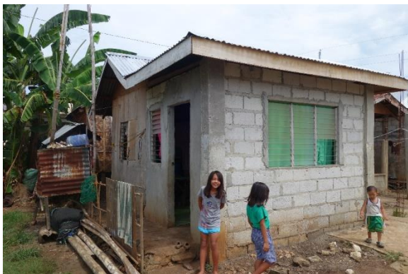
Top: Trusses used metal straps for improved strength and rafters were tied to trusses using steel wire, in addition to cleats.
