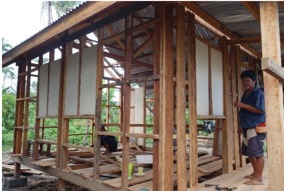
Construction of shelter walls.
