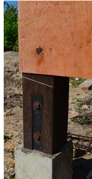
New foundations and post straps were several improvements laid out in the Shelter Cluster '8 key messages.'
