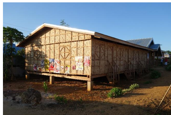
Transitional bunk house to be used while permanent houses are constructed.
