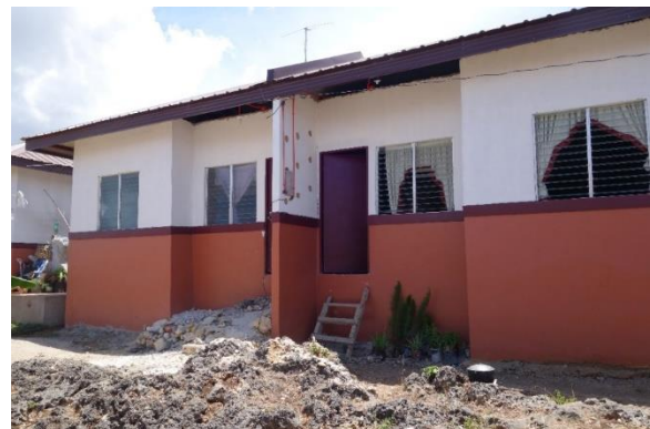
Top: Uncompleted units scatter the site pending completion due to delays.
