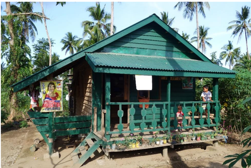
The incorporation of covered, open air spaces into shelter designs allowed for more livable conditions that increased beneficiary satisfaction.
