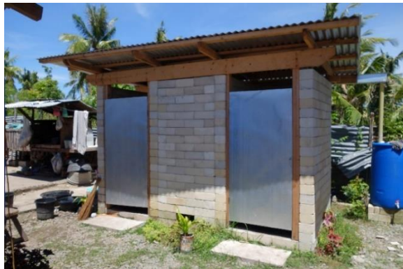
Top: An original shelter is shown. Each beneficiary was able to choose their own paint color.
