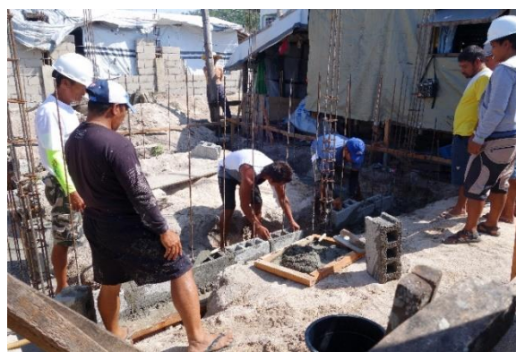
Demonstration training for block laying.
