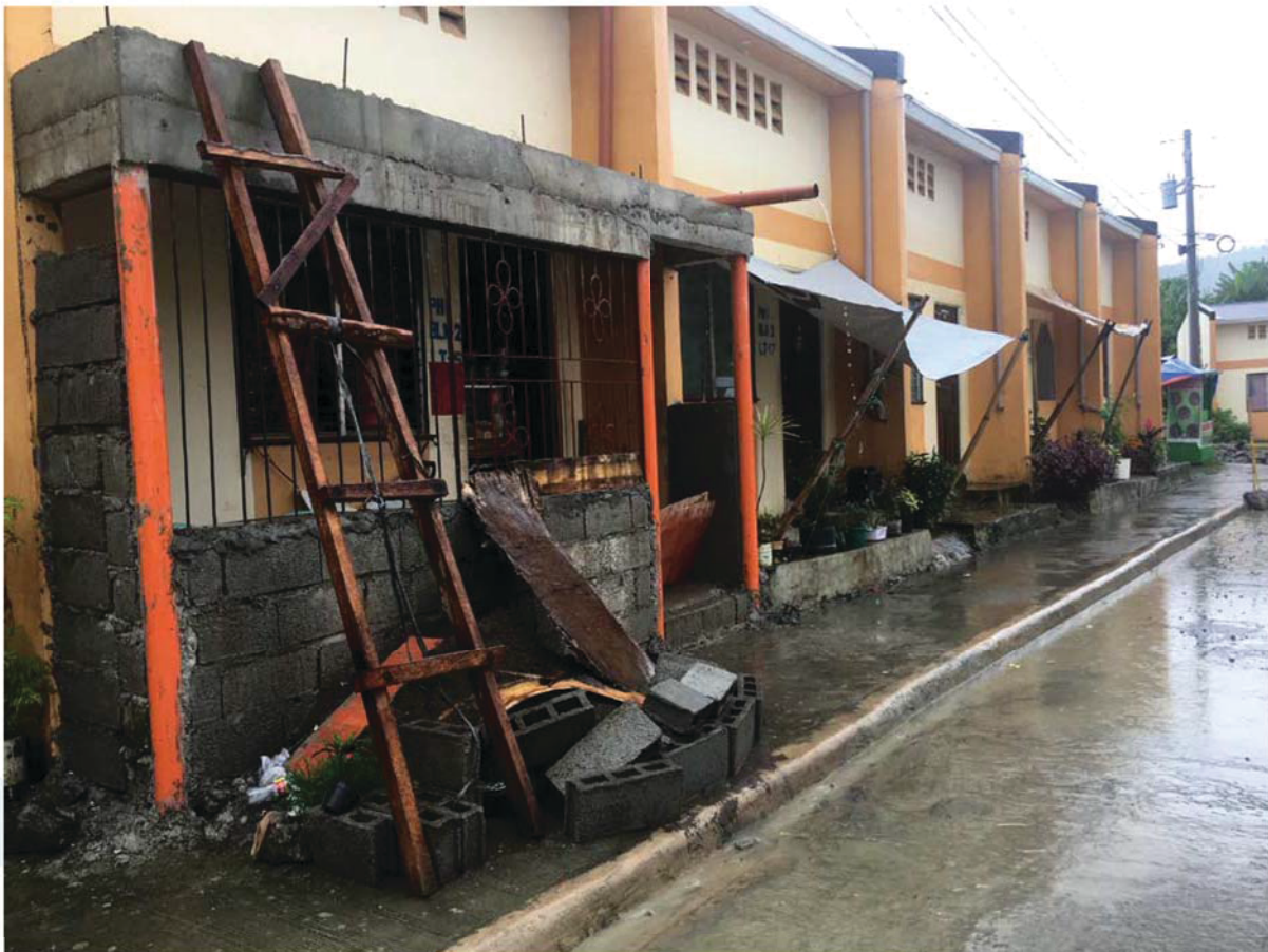
Figure 2. Household construction of a front porch
