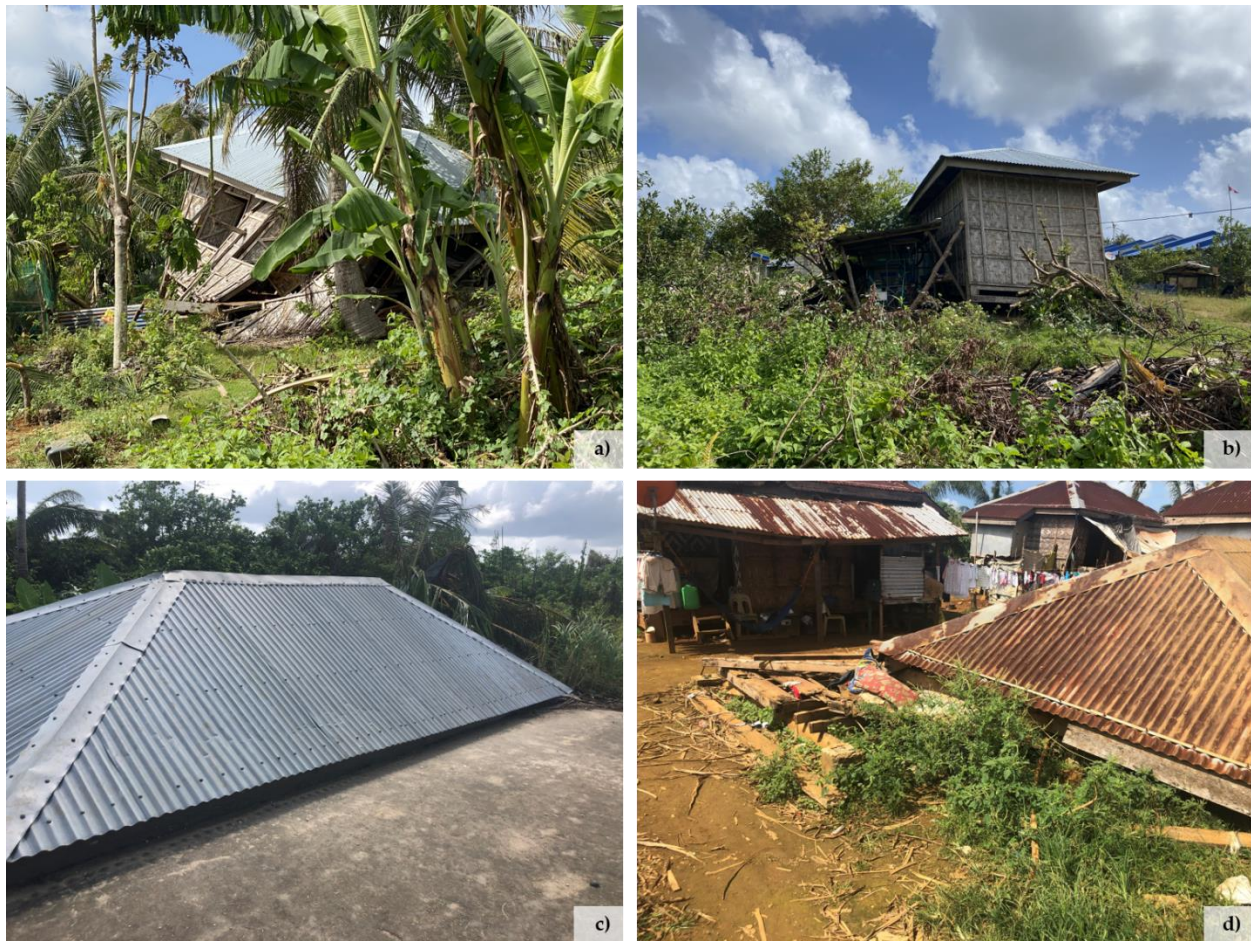
Figure 12: Examples of shelters that experienced wall failure due to failure of the column-foundation connection. a-b) Wall racking led to tilt and partial collapse. c-d) Wall racking led to complete collapse with roofs landing on the shelter. (Photos a & b by Abbie Liel).
