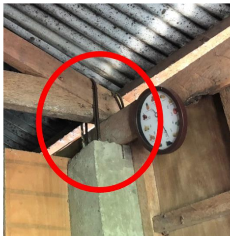
Figure 13: Example of wrapped rebar connection.
