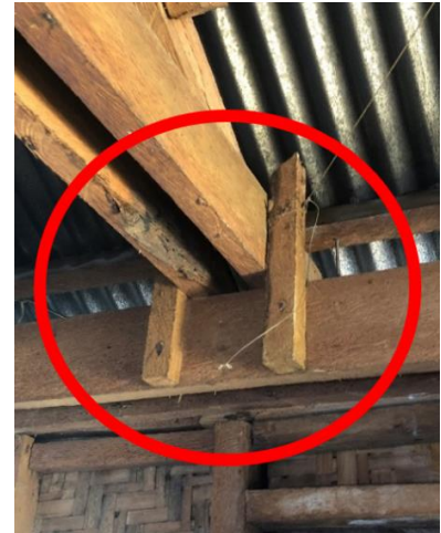
Figure 11: Truss-wall connection in Community C wooden shelter.
