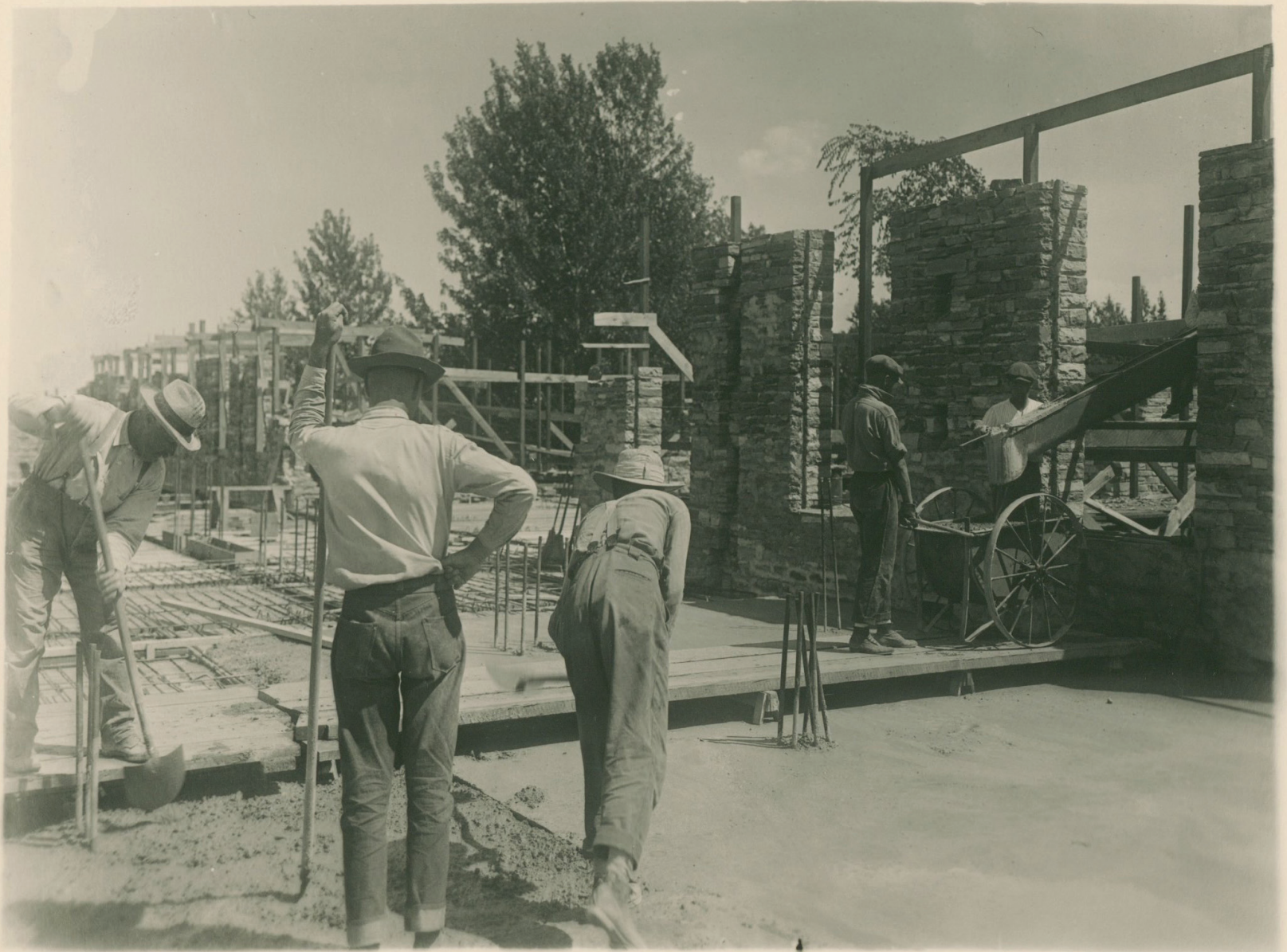
Construction of Hellems, 1921
