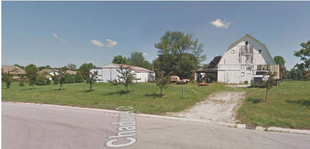
Fig 3.2.3 Fairfield Farms Barn (Google Street View)
