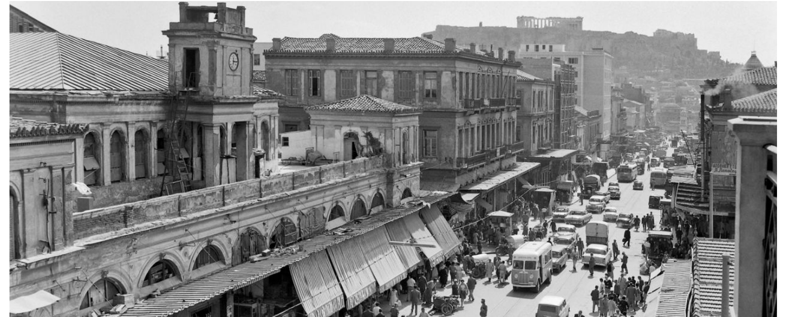
Figure 12. Decaying pre-war building stock in Athens (1949).
