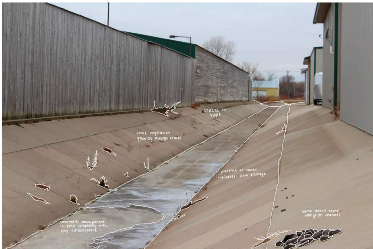
figure 33: water flows into drain from long, linear channel at edge of airport property
