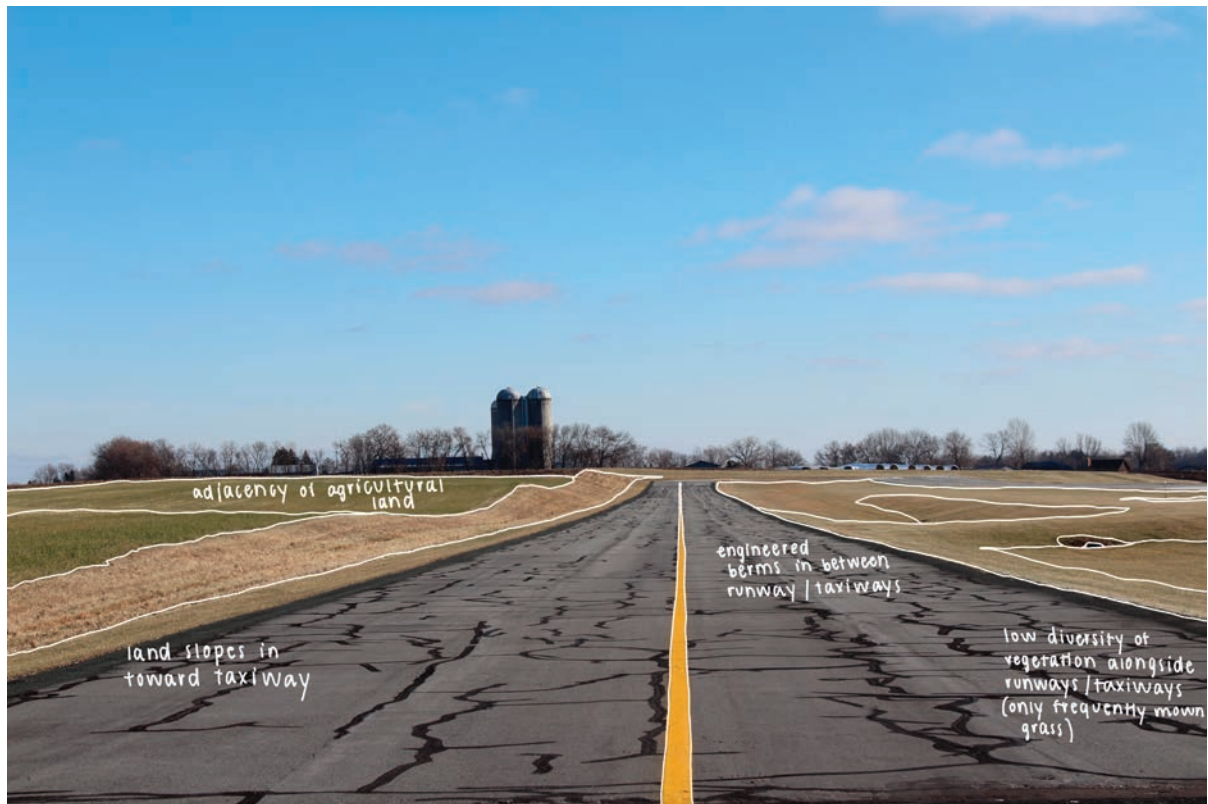
figure 38: engineered berms run alongside runway, some sloping toward the runway and some sloping away from the runway
