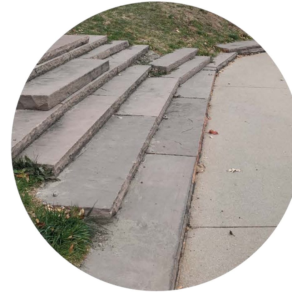
Amphitheater: Set stone slabs
