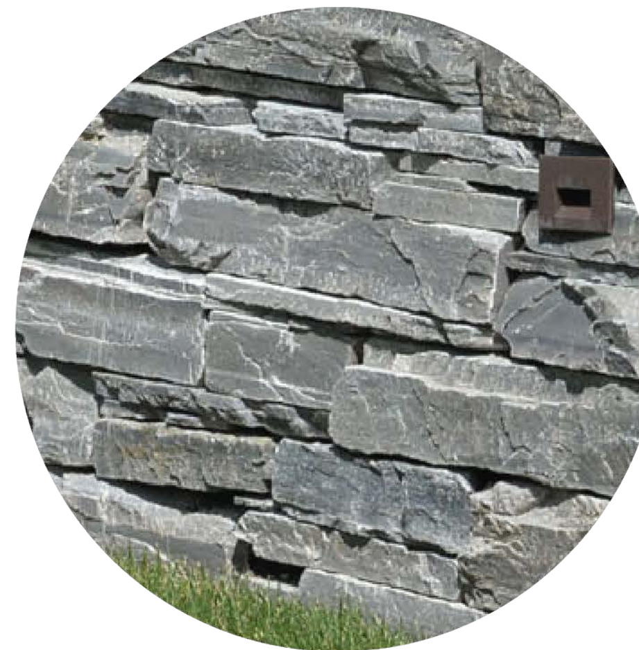
Retaining Wall: Silver quartzite
