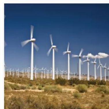
Systems and Controls
