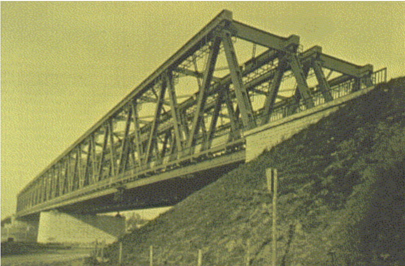
Warren Girder and Warren Truss bridge (1848)
