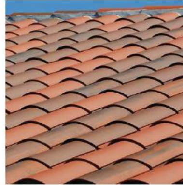
CLAY TILE ROOFING
