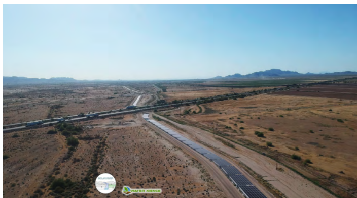
Casa Blanca Solar-Over-Canal: Phase 2. Photo courtesy of the Gila River Indian Community.
