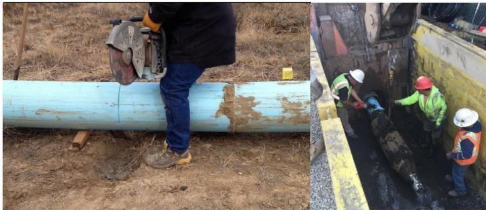
Figure 7.2. Two examples of a properly supported pipe alignment on both sides of the cut to be made.
