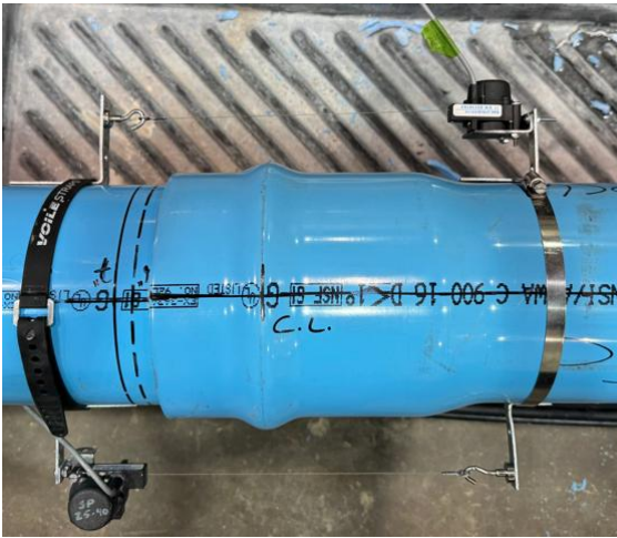
Figure 4.20. PS49 joint before testing
