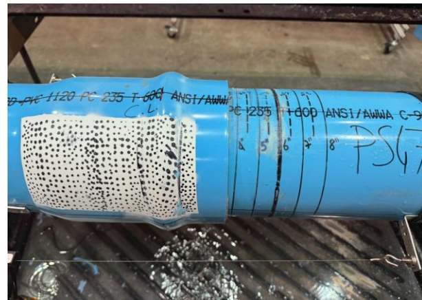
Figure 4.7. PS47 joint failure
