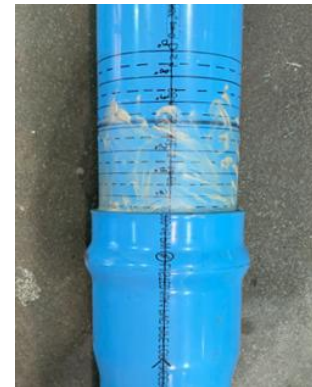
Figure 2.7. Bell and spigot before joint insertion
