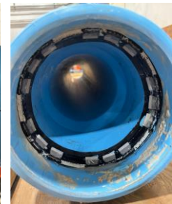
Figure 3.41. After failure for PT52
