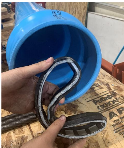
Figure 1.3. Replacing factory pipe gasket with reinforced RieberLok gripper gasket
