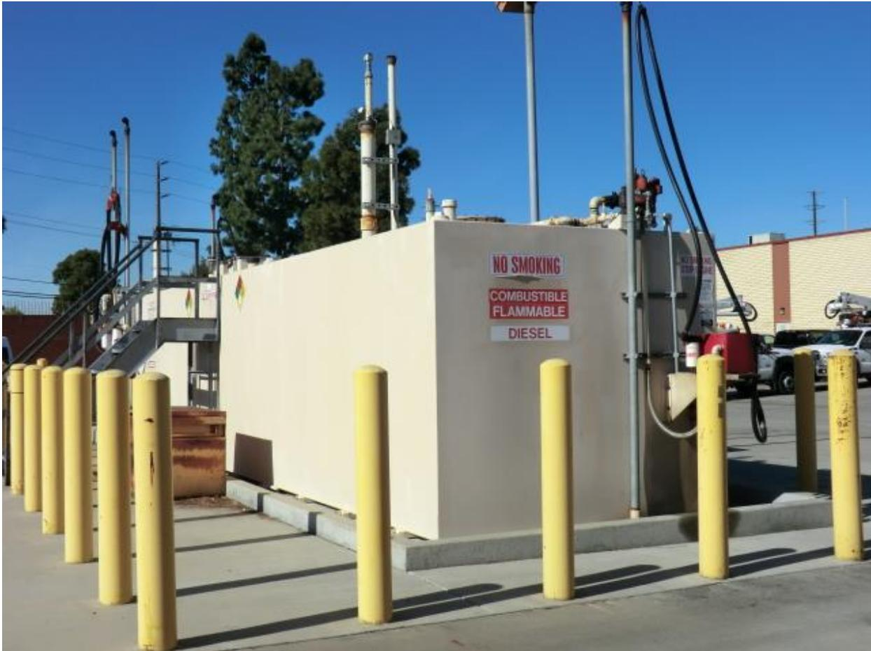
Figure 12. Above-ground petroleum tank
