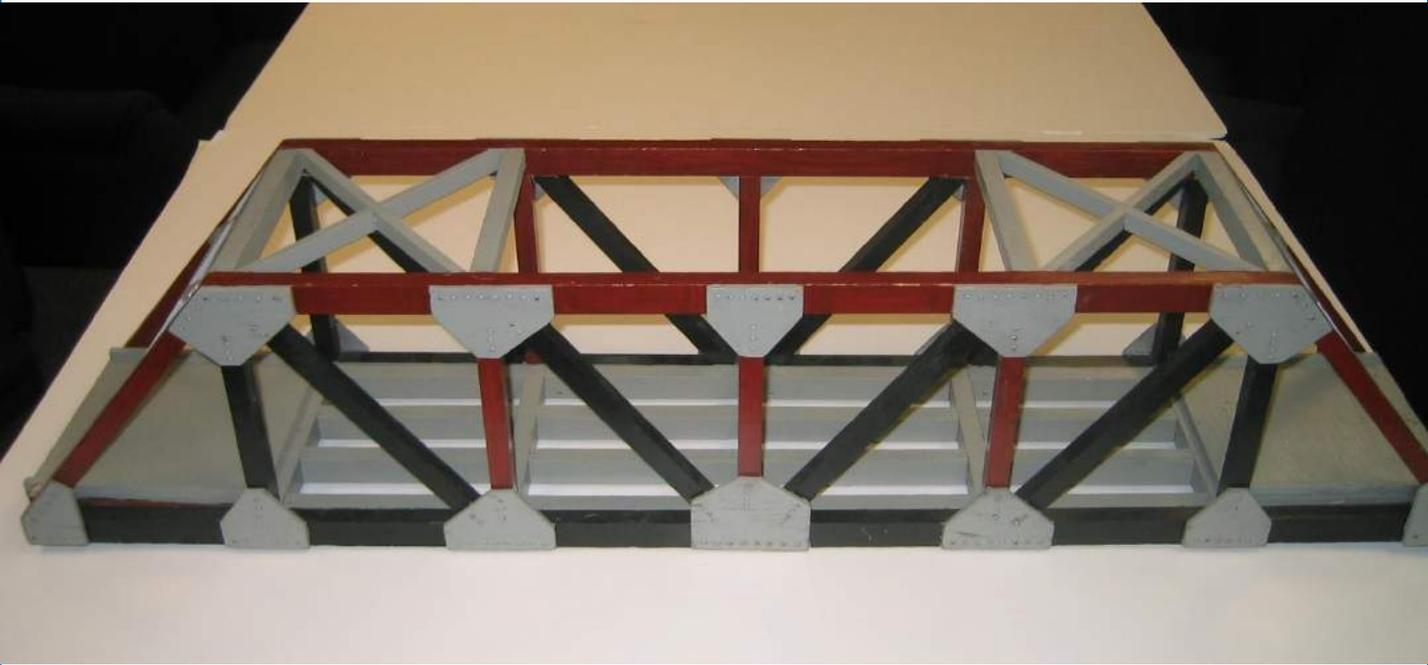
**Engineering Principle:** Bridges are more than just trusses put together. There are other important factors to a bridge that keep it stable and functional. This bridge uses gusset plates to form joints, a roadway, lateral supports to keep the trusses vertical, supports on both ends, and even curbs. It is also strong enough to hold real loads on its roadway.
