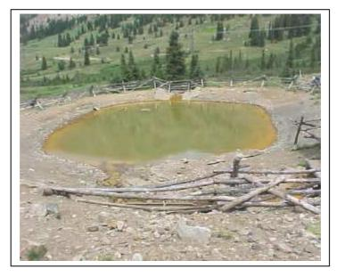
FIGURE 3.3: Holding pond at the Pennsylvania Mine. Runoff was collected and routed through this pond, which quickly saturated, in a failed remediation attempt.
