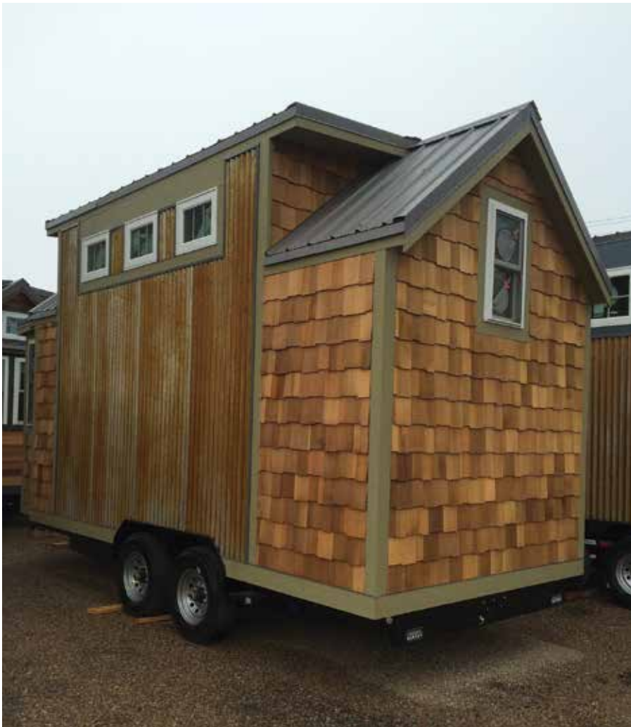
Sprout Tiny Homes built in La Junta's industrial park. Photo by Diane Graham.
