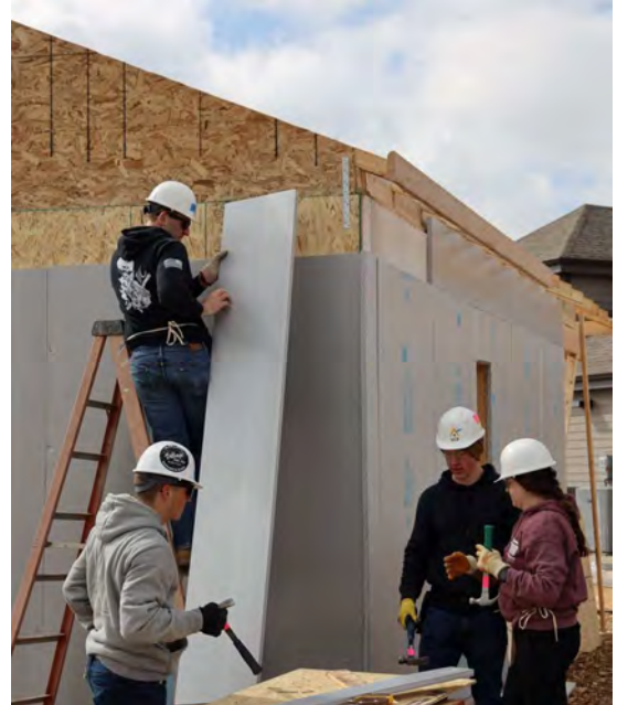
ACO CADETS AFFIXING THE “BLUE BOARDS” TO THE EXTERIOR OF A TINY HOME.
