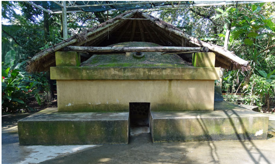
Figure 3. The Temazcal replica. It is located in the public access area of the archaeological park so people can enter it and experience the acoustic phenomena. The interior floor is the extension of the exterior bench. The front wall, above the bench and entrance, is 3.75 m wide and 1.18 m high (including it extending up, inside of the 28 cm high cornice). Photograph by Sheets.
