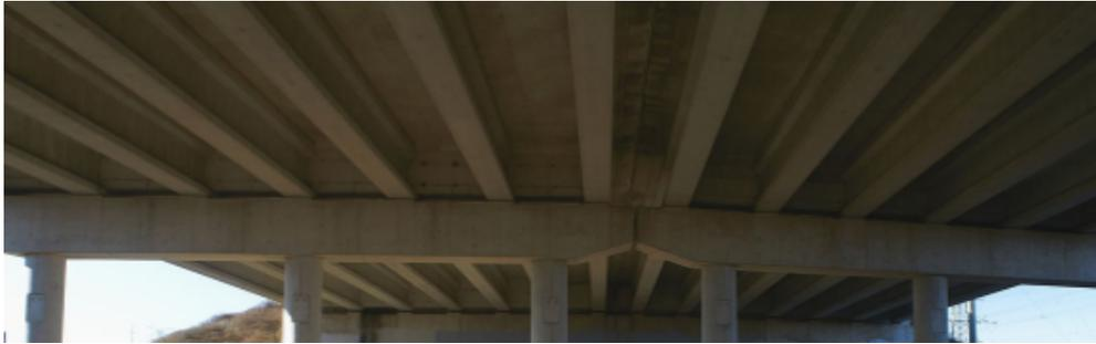
Figure 73: Longitudinal Beams along Underside of Highway Bridge (Source: Getty)
