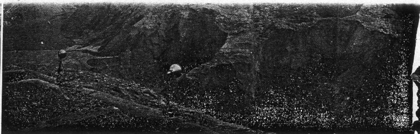
FIG. 6. Slide area following the disaster is seen from right dam abutment. Note wave-scoured area at right. Holes, or funnel-like craters, appeared in the slide as it underwent adjustment. Damaged
