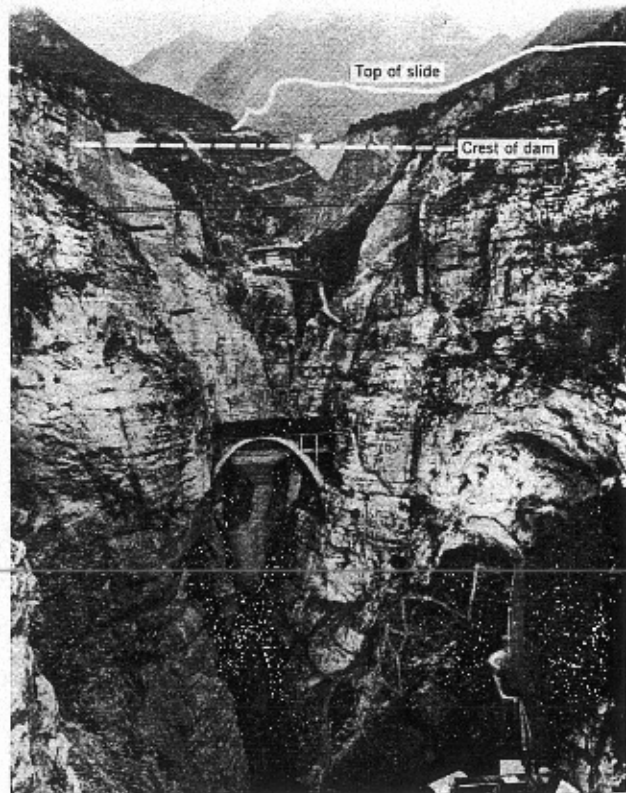
FIG. 3. Vaiont canyon is seen looking toward the reservoir site during early construction and stripping of abutments. Terrain of 1960 and 1963 slides is shown at right, with the steep cliff of Malm formation. The overtopping flood wave scoured the abutments above the dam, destroying the aqueduct and bridge (black) and stripped away the highway, lower right. Photo courtesy of Water Power.
