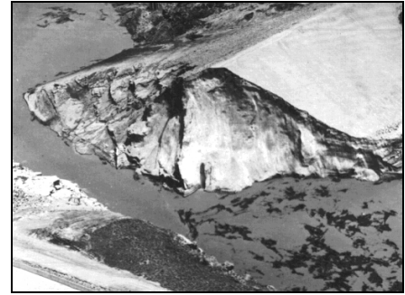
Teton Dam, Idaho failing by internal erosion on June 5, 1976. Left, initial breakout of seepage on face of dam. Middle, wave pouring through eroded opening. Right, after wave passed through.
