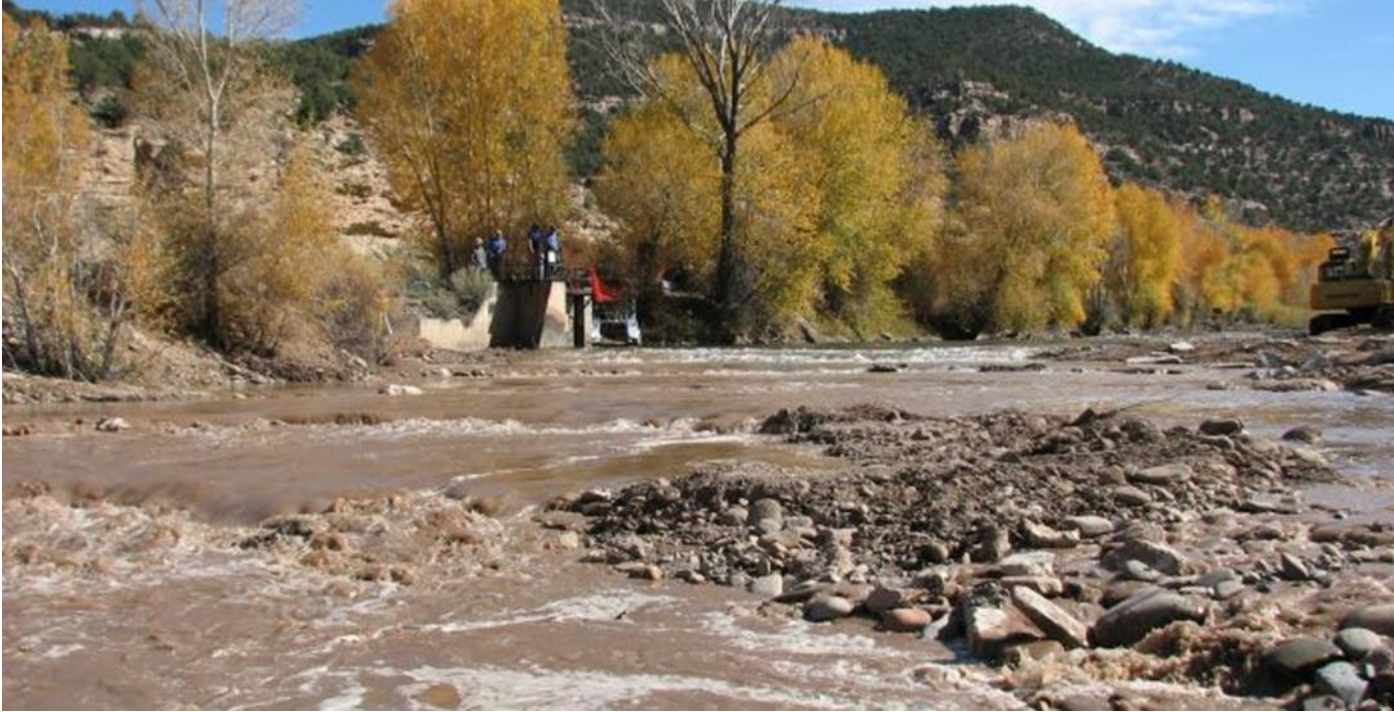
The San Miguel River flowing over the CCC Ditch check structure | Scott Hummer
