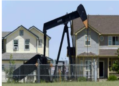
Fig. 3. Pump jack next to homes in Frederick, CO. 238
