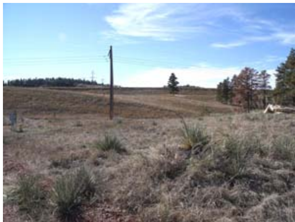
An 80-foot-high containment wall for a coal-ash storage pond blends into the landscape near the Colstrip plant. Photo by Kristen Lombardi.
