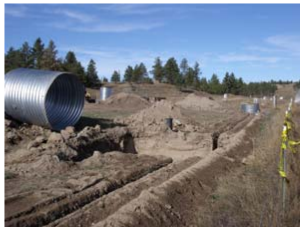
A Colstrip construction site where new recovery wells are being installed. Photo by Kristen Lombardi
