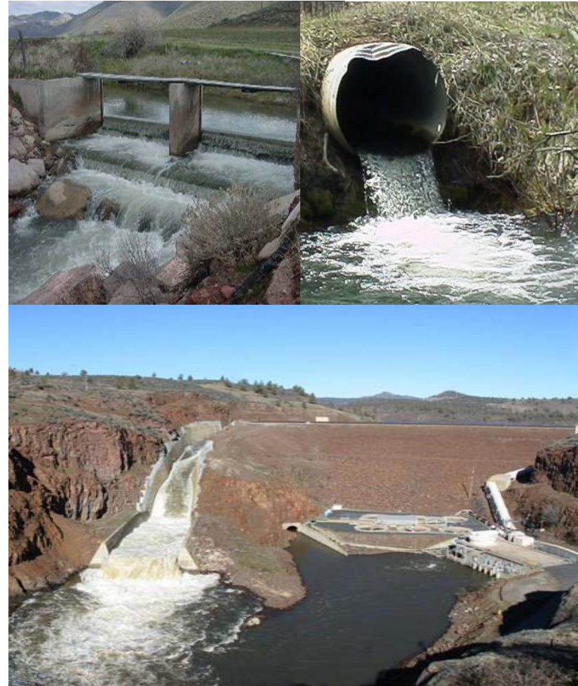
Diversion Bear River ID and a perched culvert Iron Gate Dam, Klamath River CA
