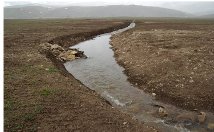
After: the water has started to flow
