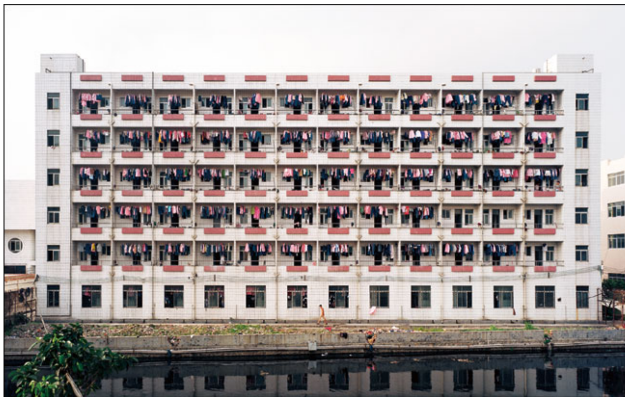
A workers' dormitory in Dongguan District Gaobu Town, China.
